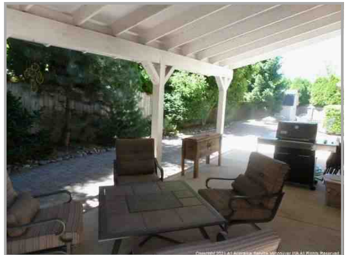
Rear Covered Patio, Wood Beam/Composite Roof
