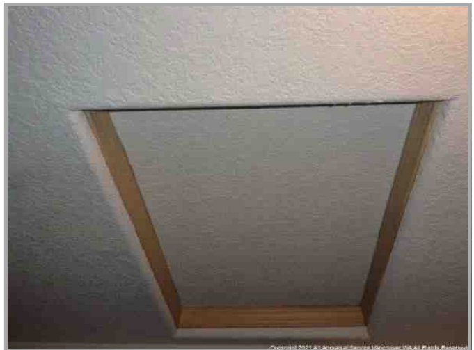
Attic/Scuttle Access (Primary Bedroom Closet ceiling)
