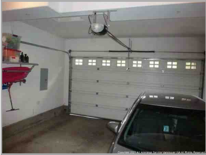
Two-Car Garage, door opener with safety sensors, finished
