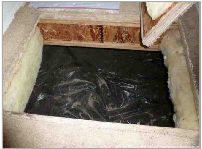
Crawlspace Access (Foyer Closet Floor)
