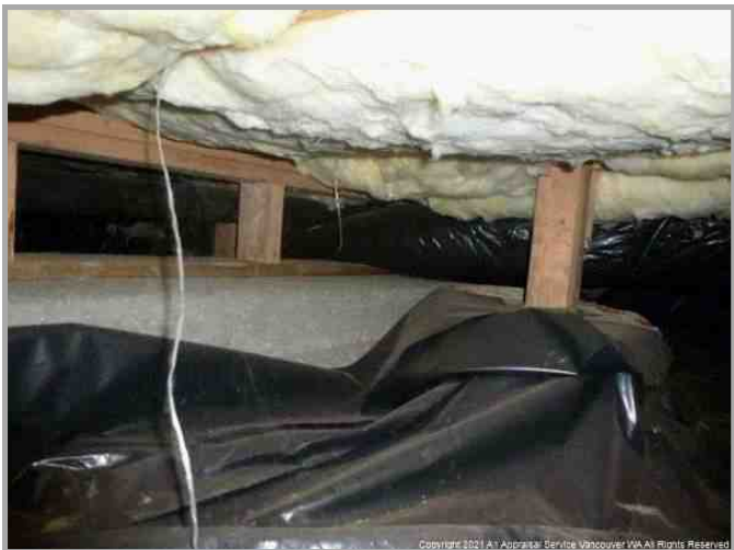
Crawlspace (head and shoulders observation only), see comment
